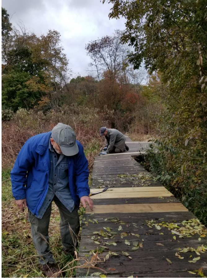
Finger Marsh Boardwalk Repairs in October
